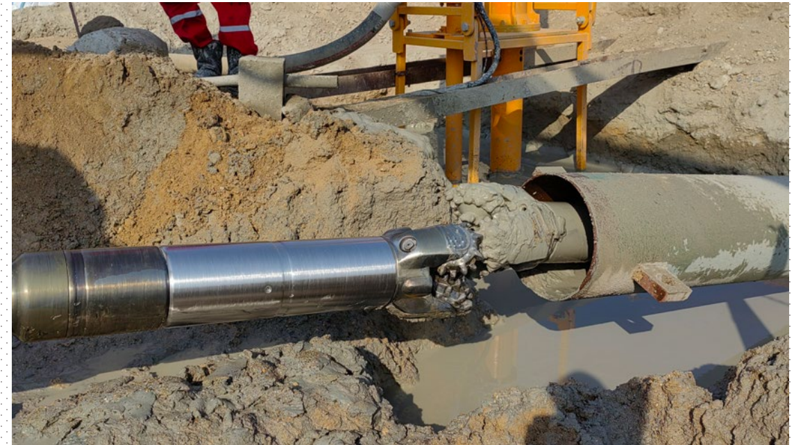
Above: Pilot hole for gas pipe successfully intersected and punched out
