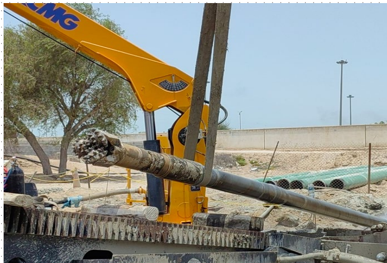
Left: Pilot hole for FOC successfully intersected and punched out
