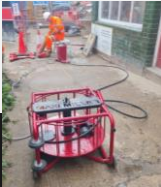
Limited access no issue, portable equipment.
