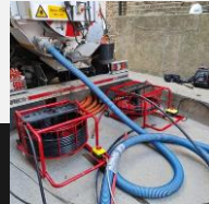
Small worksite footprint. Jetvac was used periodically to remove debris.
